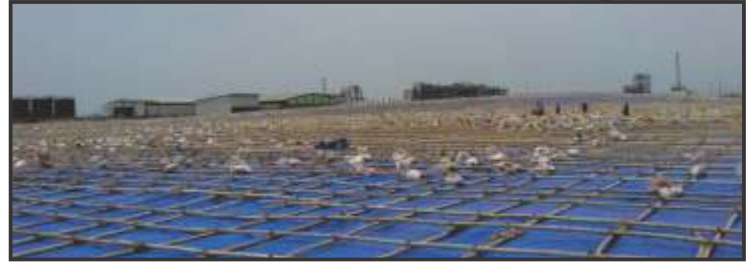
LANDFILL COVERING DURING MONSOON
